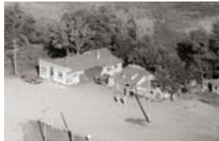
West Salisbury General Store and Post Office opened in 1911 a mile west of the Rural Salisbury School at what became known as Salisbury Corner. Peter and Annie Yohemas purchased the store from the Richardsons in 1941. The store served as a community hub; it was moved a mile south in 1964 to make way for highway expansion. (#315-33-14, Homestead Aerial Photo Ltd.)
