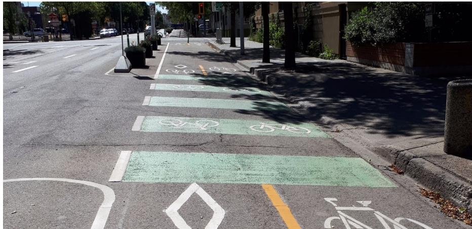
Figure 5.27: Bicycle Pavement Markings at Mid-Block Conflict Zones
