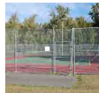
Damaged Tennis Court Fencing
