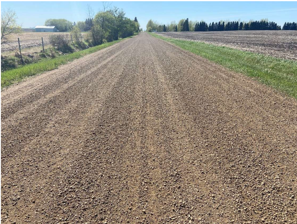
Class IV road with loose gravel surface
