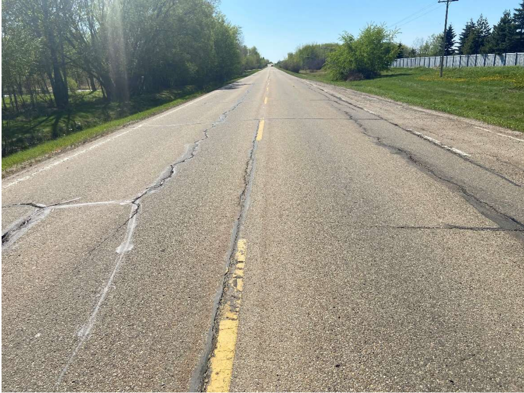
Class I road with old hot mix surface
