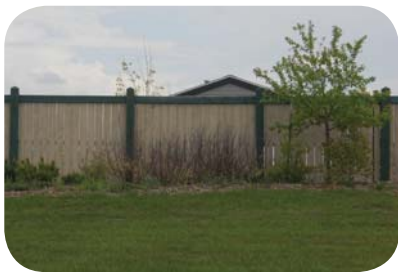
Existing Fence at Maple Ridge:
